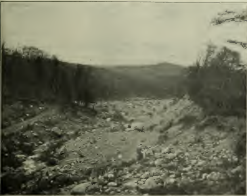
WORK OF HYDRAULIC POWER, NEAR RINGWOOD
